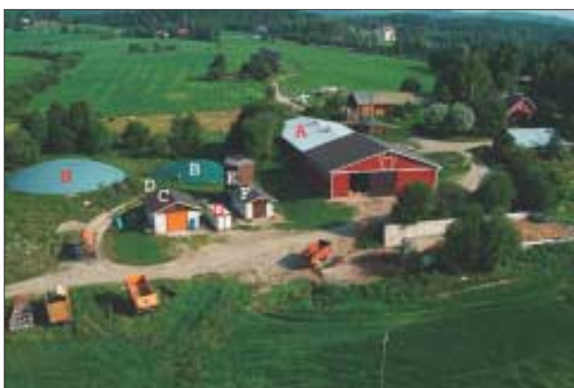
Figure 1: The Kalmari farm biogas reactor system in Leppävesi, near Jyväskylä in Finland. (Lauri Jokela)
