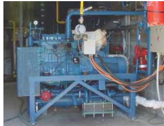
Figure 3. Micro-CHP system: 30 kWe and 60 kWt. (Jeremias Kalmari)
